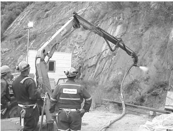
Figure 5. Robotic arm for shotcrete application.
