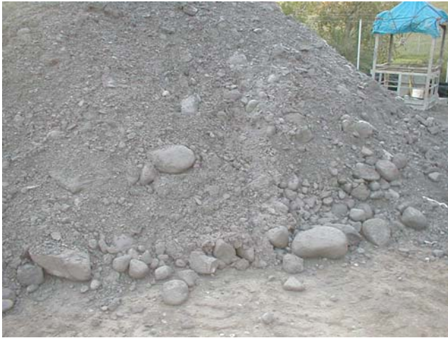
Figure 4. Excavated Soil From Frozen Shaft.
