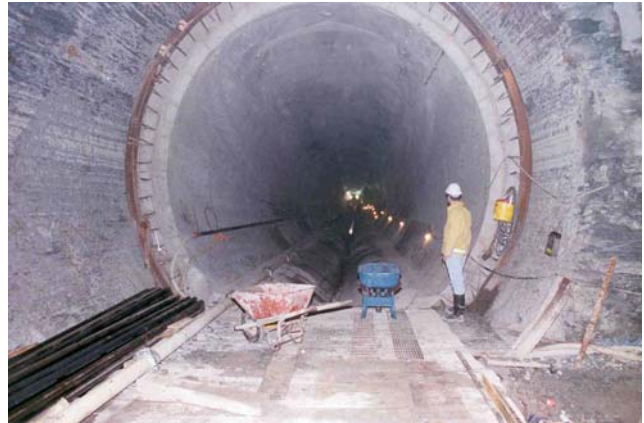
Figure 7. View of Cast-in-Place Concrete Liner– MCT-2 Tunnel.
