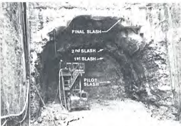
Fig.5. Portal face excavation
