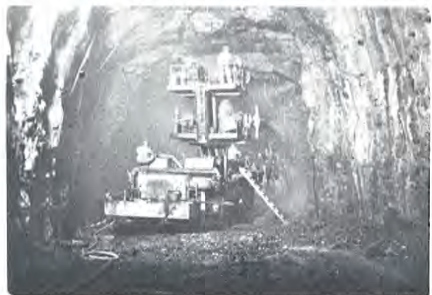
Fig.6. Full face excavation
