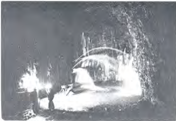
Fig.9. Zone 1, flow from drill holes
