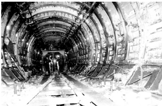
FIGURE 2 Full view of concrete form
