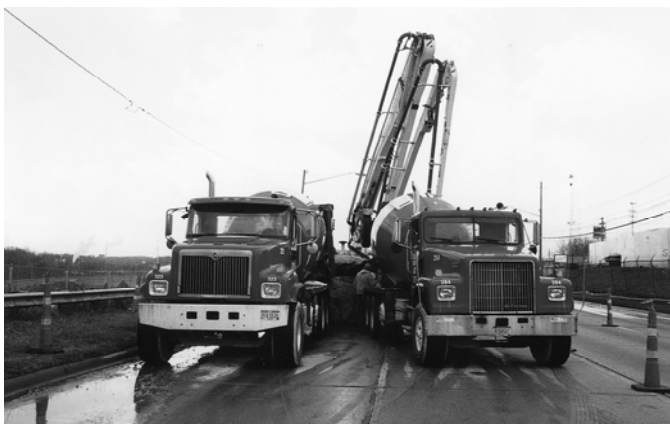
FIGURE 8 Concrete delivery at down-hole position
