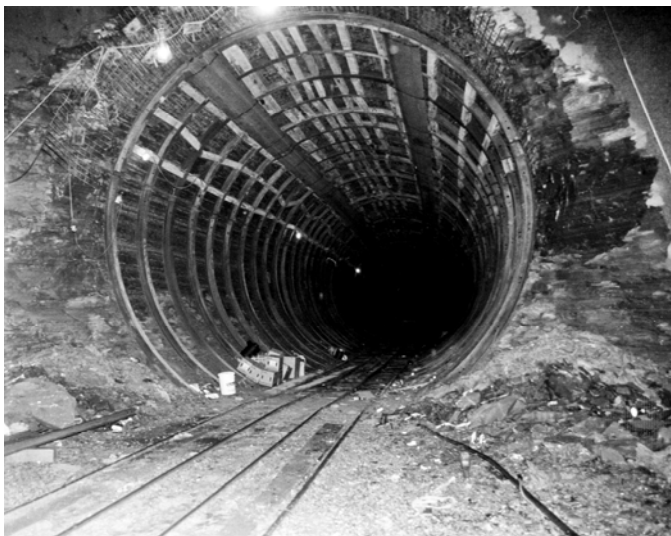
FIGURE 3 View of Z-beams and tunnel support
