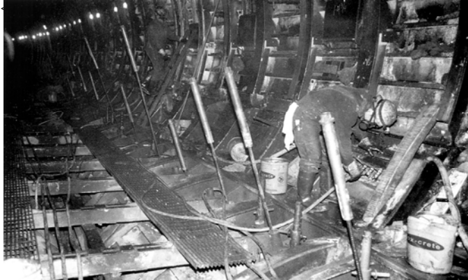
FIGURE 6 View of tie-downs at form invert
