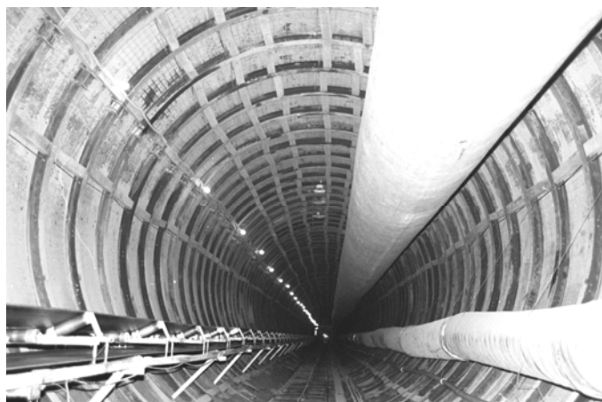
Figure 3. View of installed primary support
