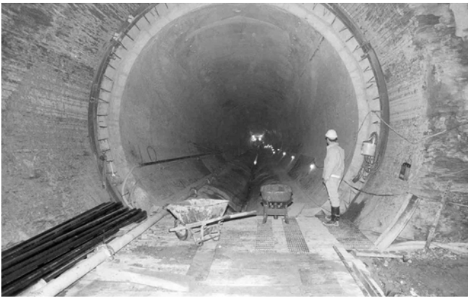
Figure 6. View of placed liner
