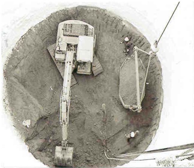
Figure 6. Soft-core soil excavation.
