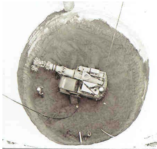
Figure 8. Mechanical trimming of frozen ground
