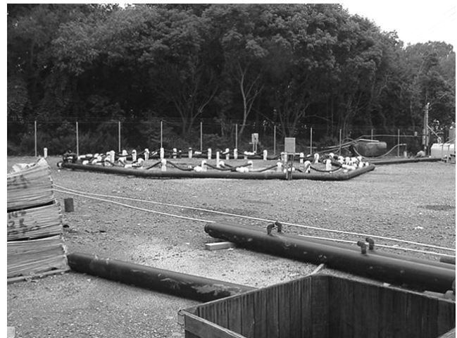
Figure 3. Freezing system layout at Shaft 13.
