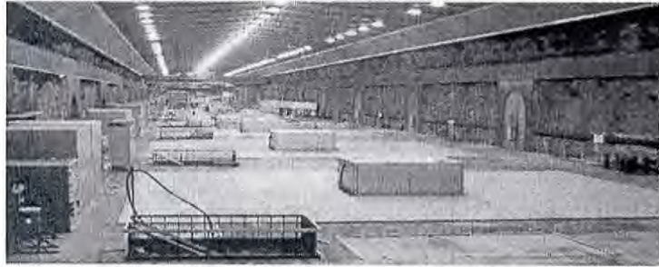
Figure 3 La Grande Underground Powerhouse, LG-2, Hydro Quebec.
