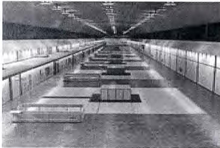
Figure 5 Churchill Falls 6500MW Underground Powerhouse
